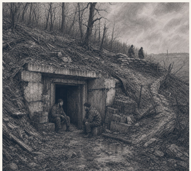
Bamut bunker mouth and wooded slope.
